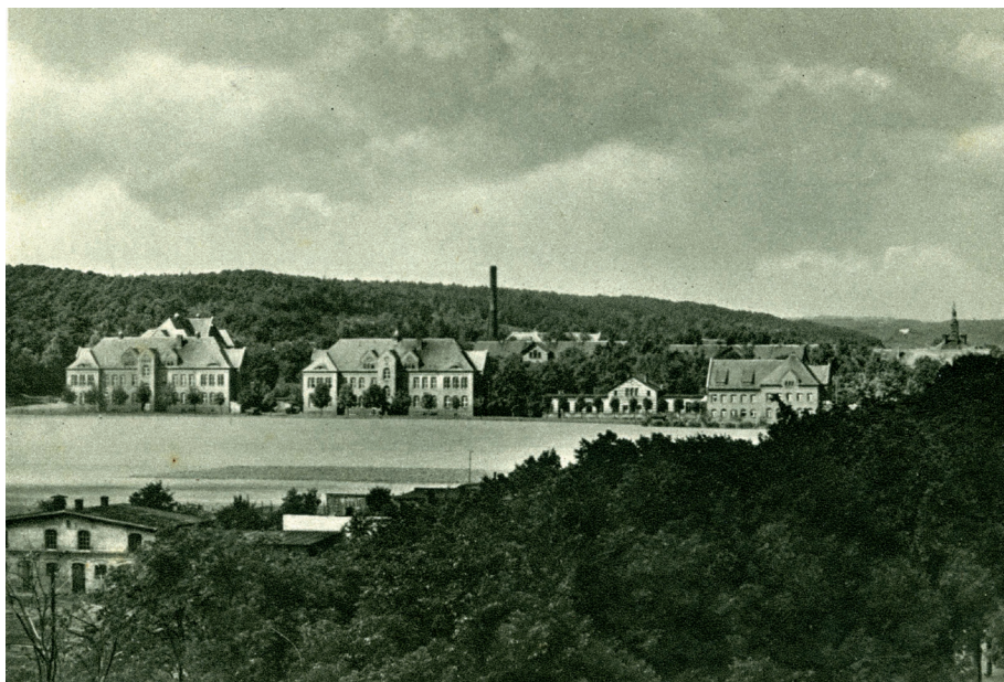
The complex of buildings where the Educational Facility for Boys in Wejherowo was situated in the years 1939–1943, now the seat of the School-Educational Centre no. 1 under the name of Janusz Korczak, the Museum of Writing and Kashubian-Pomeranian Music in Wejherowo
